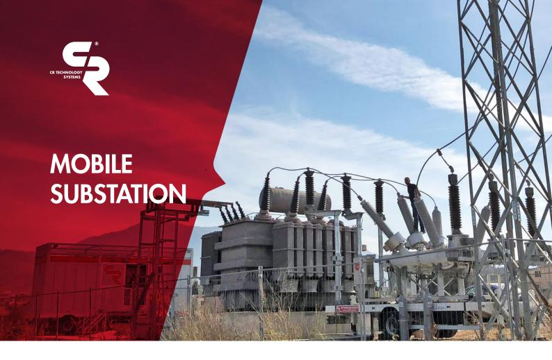
C.R. Technology Systems mobile Substation is an electrical substation mounted on semi-trailers. It's a smart solution to supply energy "in motion", with excellent performance and reliability.
